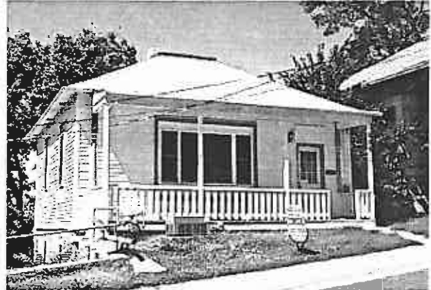
626 3rd Street – Raised Hipped Cottage
