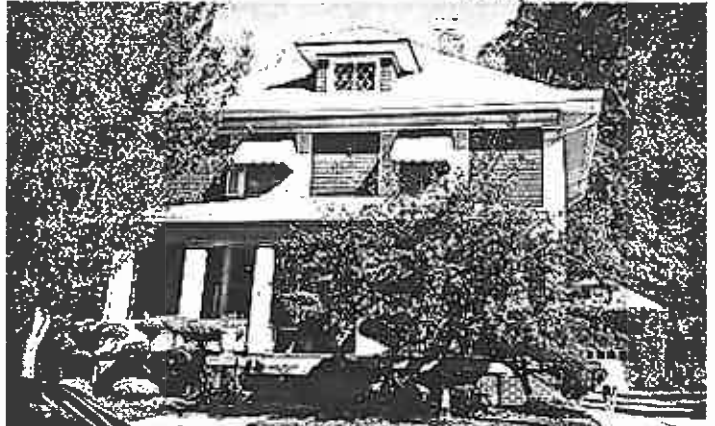
519 Clark Avenue – Foursquare
