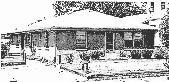
234 Bluff Street – Ranch
