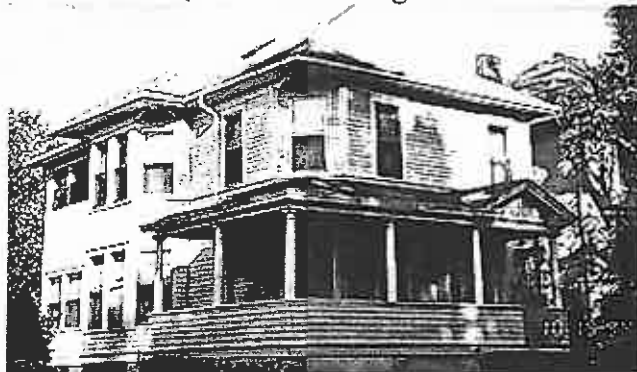
40 Bluff Street – Foursquare Variant
