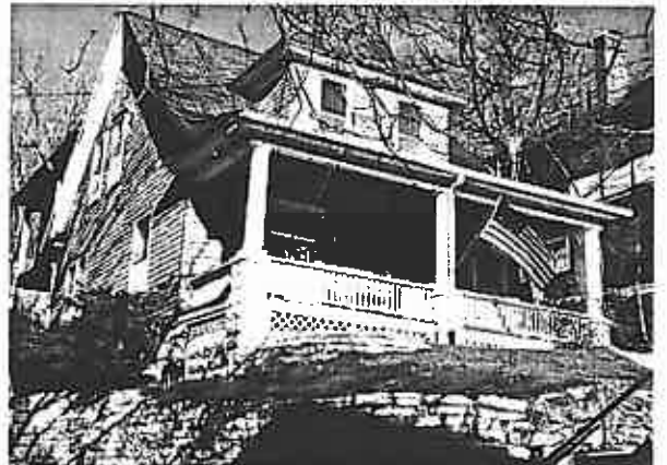
206 Turley Avenue – Colonial Revival
