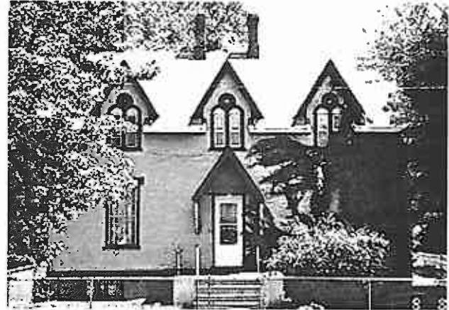
625 Bluff Street – Gothic Revival
