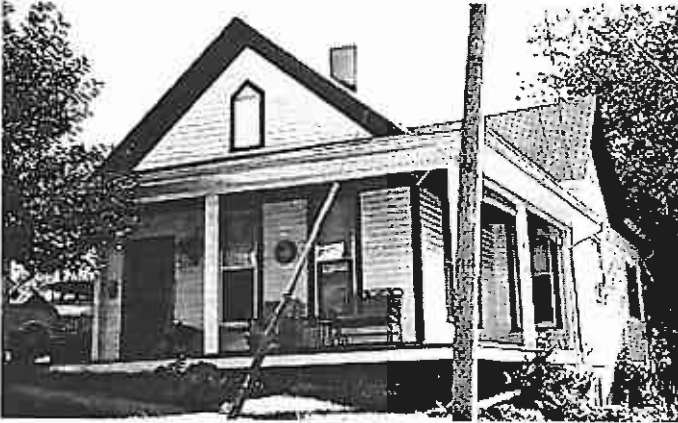
225 Fairview Avenue – Greek Revival Cottage
