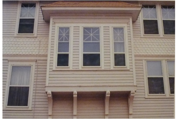
Window detail from the north and south sides of the house
