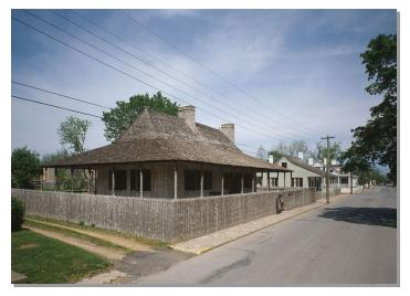
of these Creole houses are *poteaux en terre* (posts-in-the-ground) where the walls made of upright wooden posts. In addition, these posts do not support the floor of the home. The floor is supported by separate stone pillars. Set into dirt, the walls of such buildings were vulnerable to flood damage, termites and rot. This risk, however, could be mitigated by the abundance of white oak which has some resistance to these dangers.
