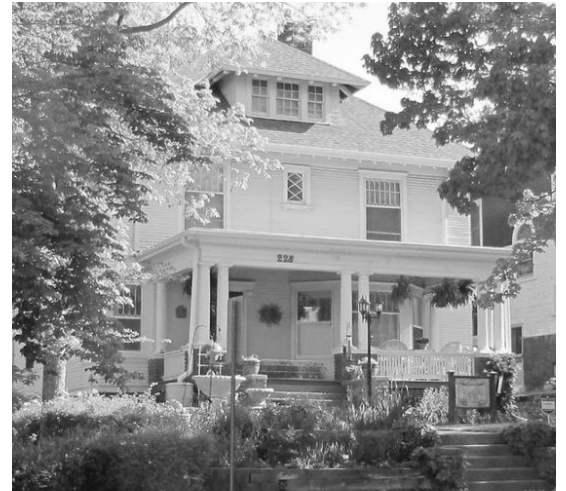
The Charles T. Officer home, located at 228 5th Ave., features narrow clapboard siding, a hipped roof with eave overhang and hipped dormers with exposed rafter
