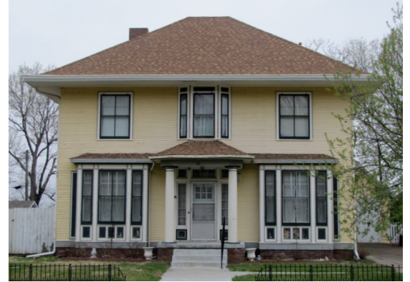
The John P. Hess House, 36 Bluff Street
